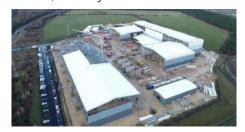
The converter stations transport and convert energy via a cable known as an interconnector. Construction of both converter sites is well underway. They are being built by ABB and use high-voltage direct current (HVDC) technology, which has been specially designed to transmit power underground, underwater and over a long distance.
