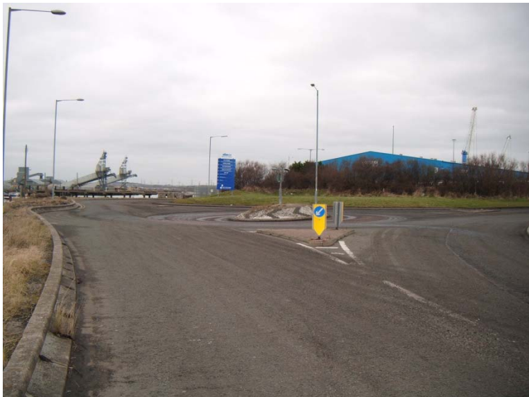
Plate 14.4 Port Access Roundabout Junction
